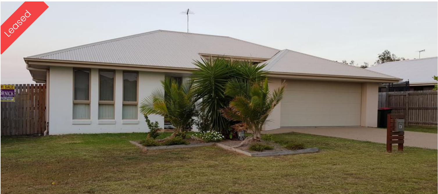
7 Florida Crescent, Parkhurst
